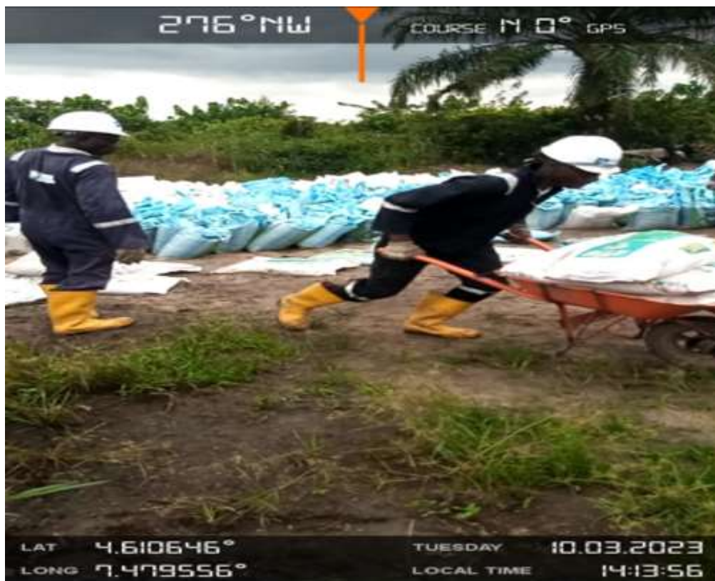
Plate 2: Movement of Sandbags to Biocell Ongoing
