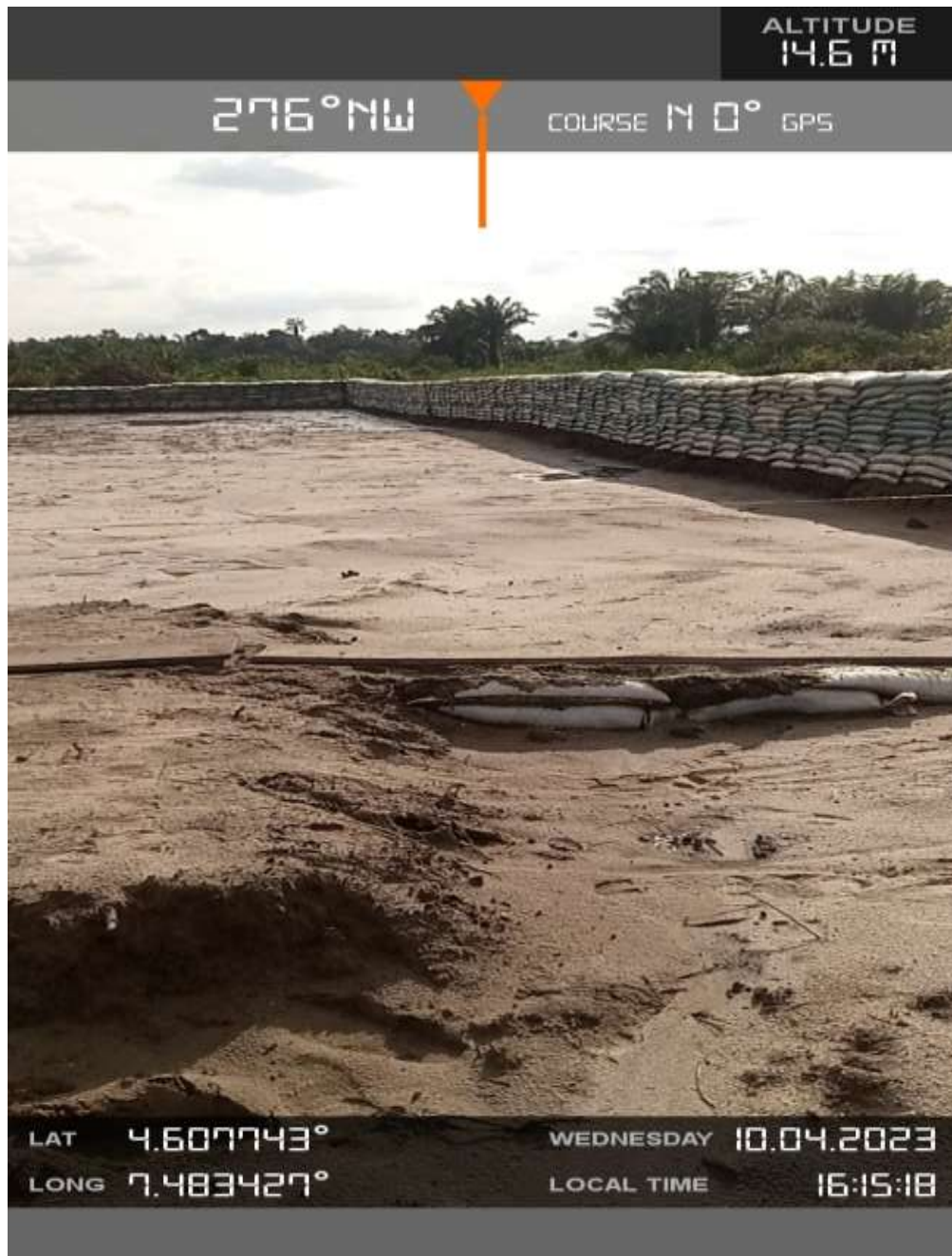
Plate 5: Cross Section of Stacked Sandbags
