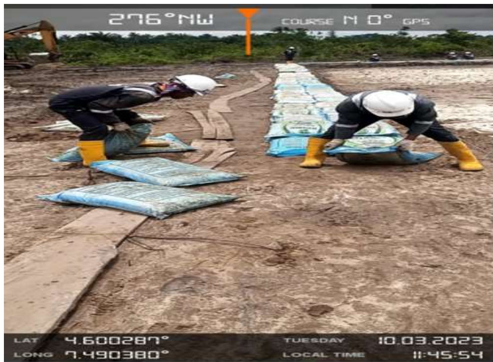
Plate 3: Laying of Sandbags
